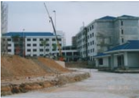
View of the ESSET Complex while under construction
